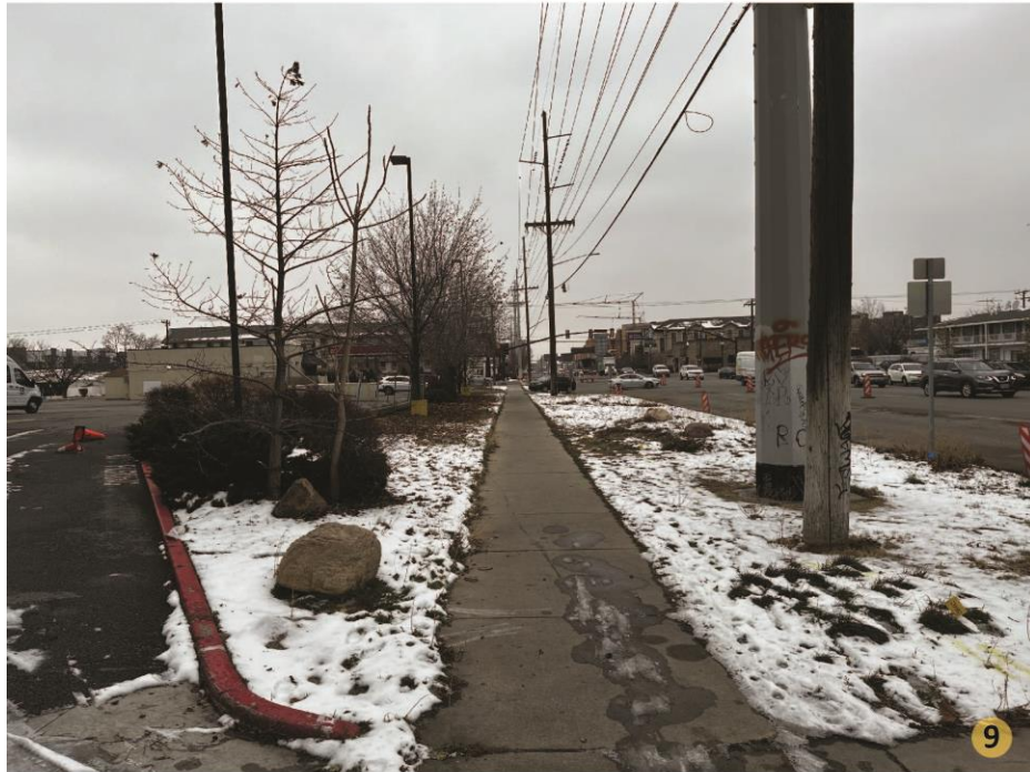
600 SOUTH Looking West
