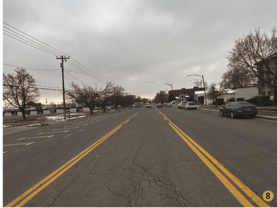
200 WEST Looking South
